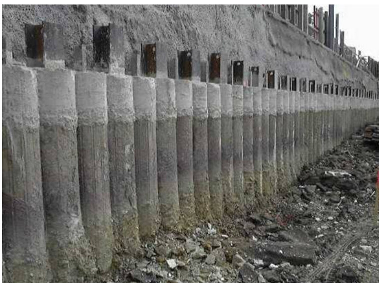
Secant pile wall after excavation.
