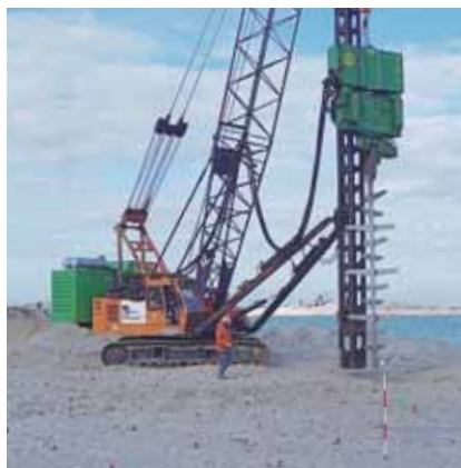
"Vibrowing" compaction of sand in an area sensitive to settlements.
