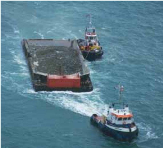
Dredged material being towed to the reclamation area.
