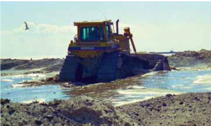
Sand from borrow areas was brought to the island for the construction of portions of the traffic corridor.
